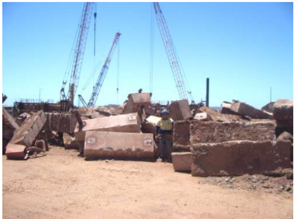
Figure 2. Concrete conveyor footings at the Rio Tinto worksite in Dampier.
