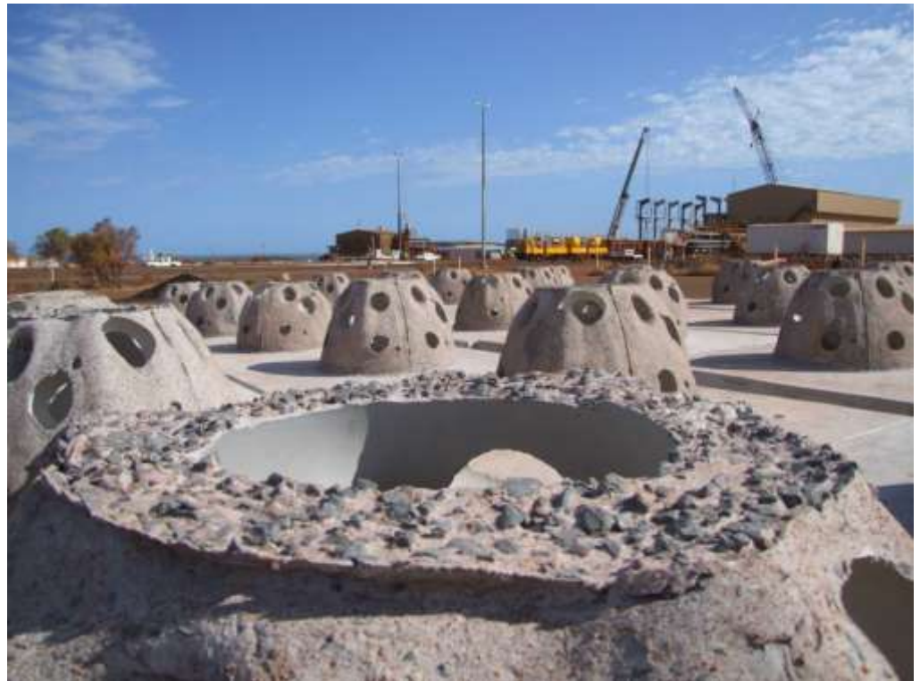
Figure 1. Recently constructed concrete ReefBalls at the Rio Tinto worksite in Dampier.
